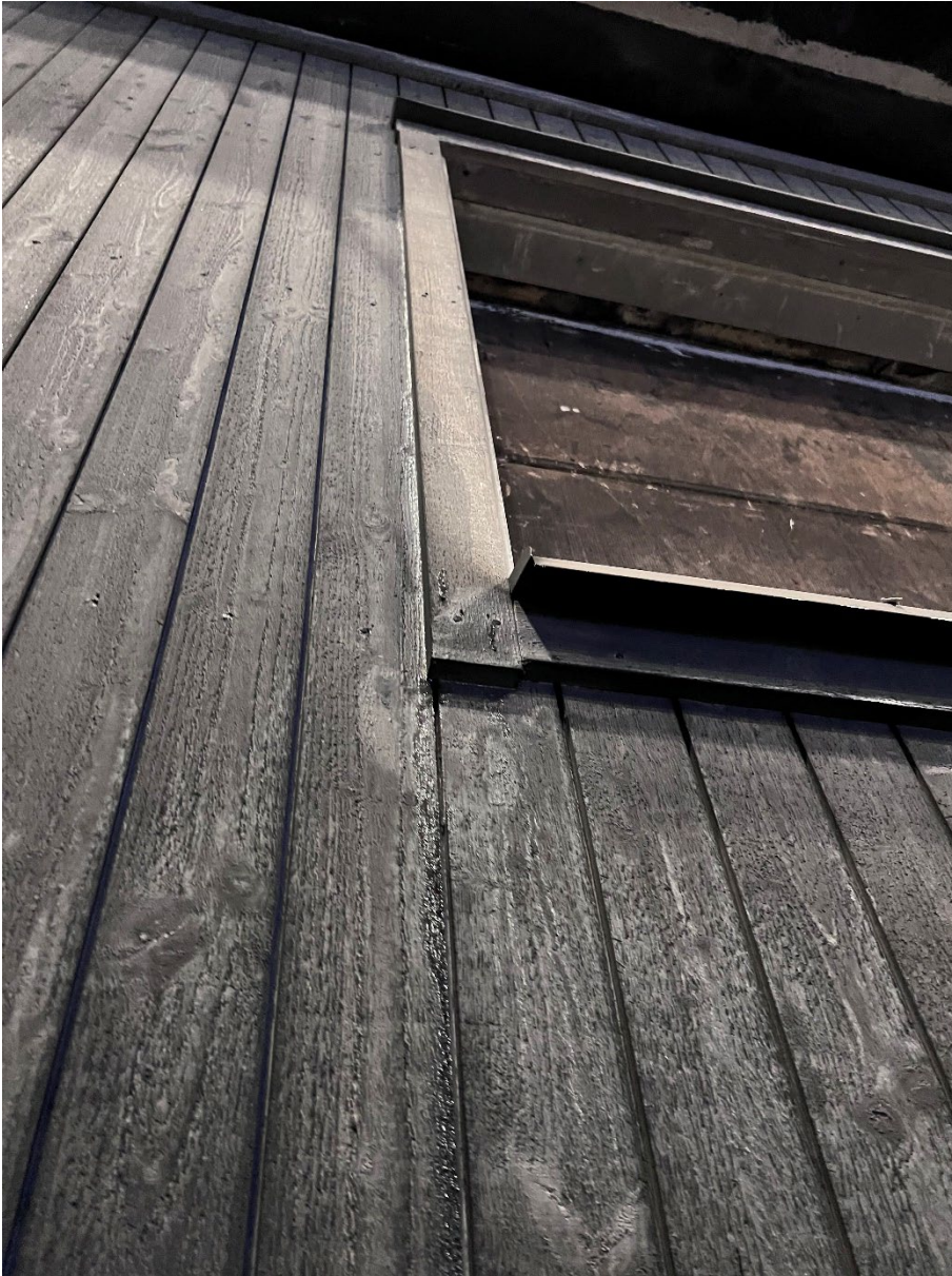
Photo A- 4 Close up of the upper part of the test specimen after the test.
