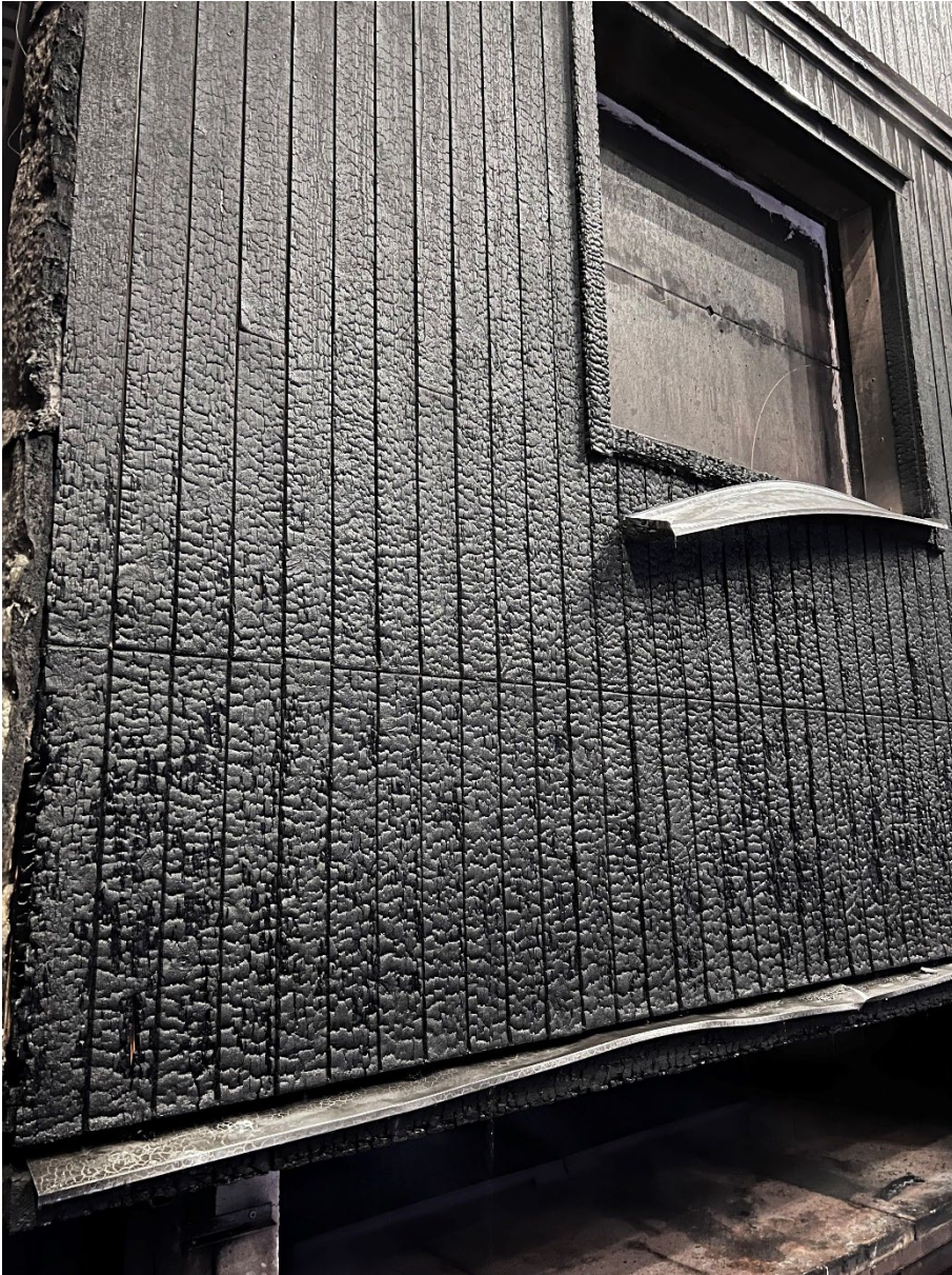
Photo A- 3 Close up of the lower part of the test specimen after the test.
