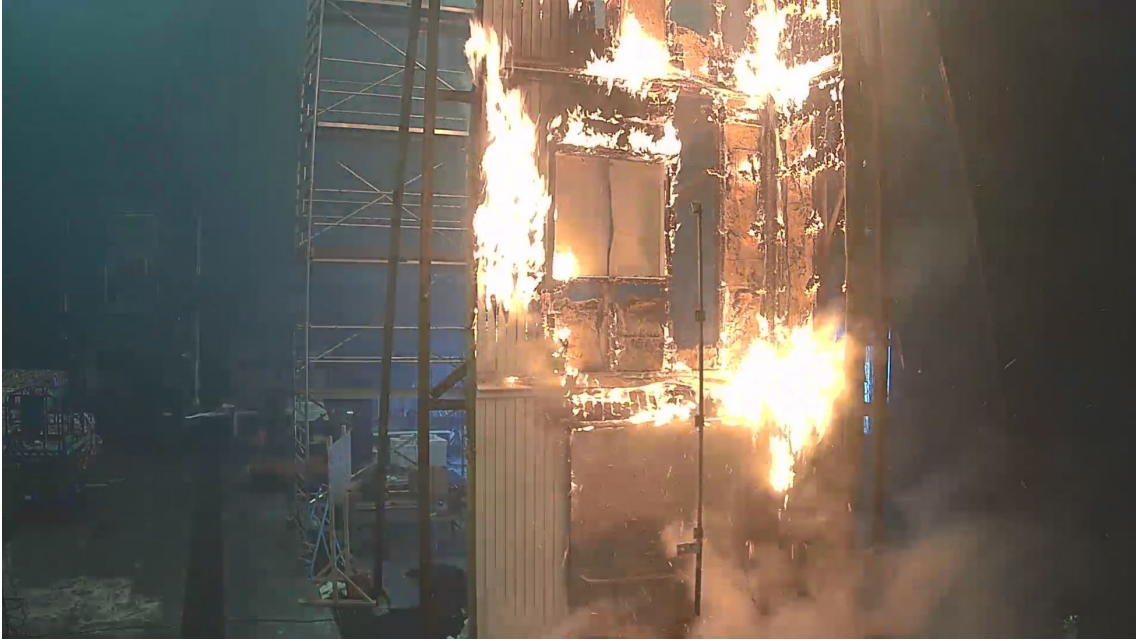
Photo 23 Draft proposed European test method, 32 minutes after first flames emerge out of the combustion chamber and 3.5 minutes after the wood crib was extinguished with water.
