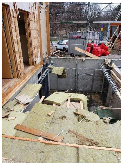
Figure 21 - Basement floor in concrete with storage rooms and laundry rooms.
