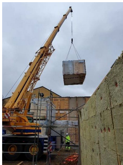
Figure 16 - After detaching the modules, they are lifted down using a crane.
