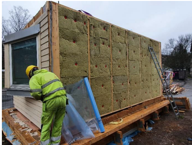
Figure 17 - The modules are covered with plastics before transport and intermediate storage.
