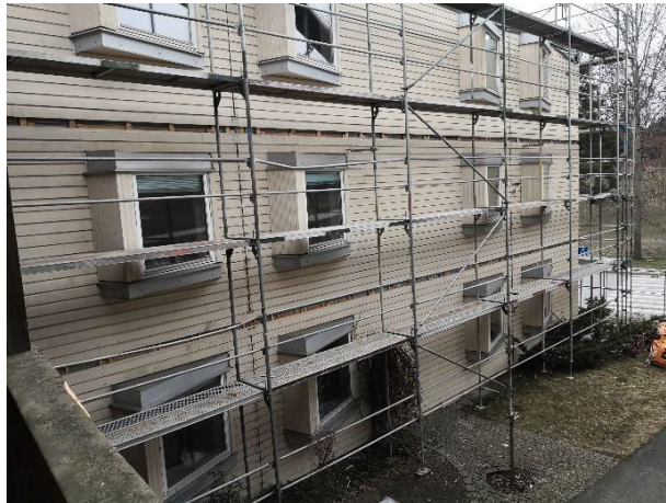
Figure 10 - Apartment modules from the outside.
