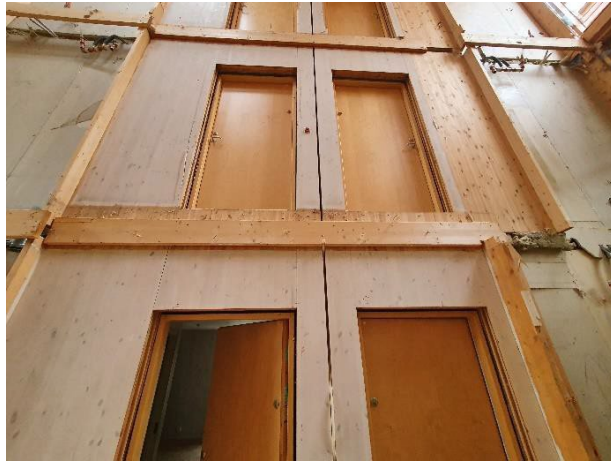
Figure 11 - Apartment modules from the inside.
