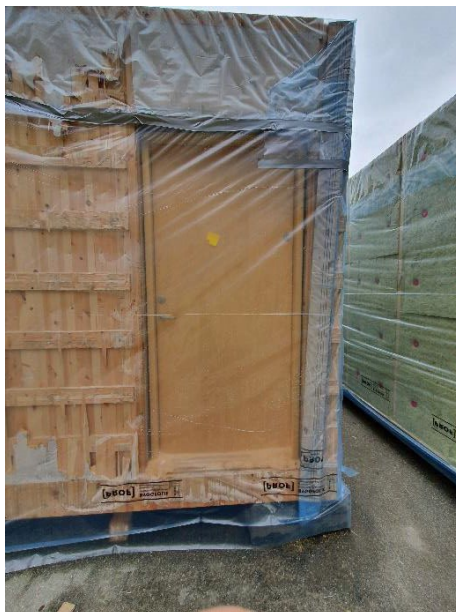
Figure 19 - Risk of moisture problems when the modules are covered with plastic (already condensation on the inside).
