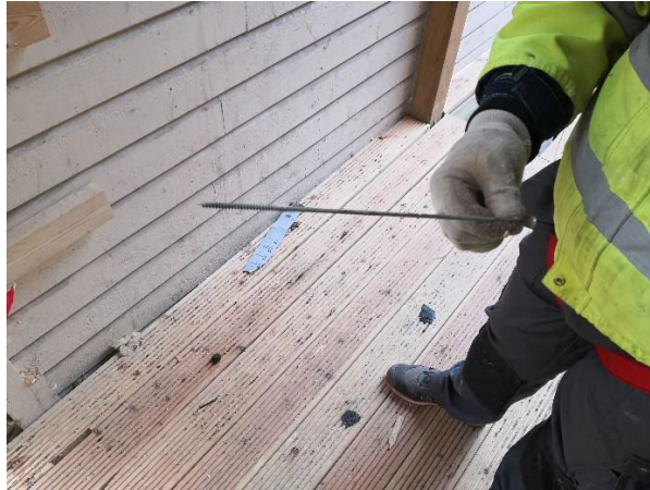
Figure 14 - Example of long screw, used when the modules were screwed together.
