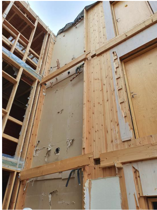
Figure 3 - Transition between module and access balcony/staircase.
