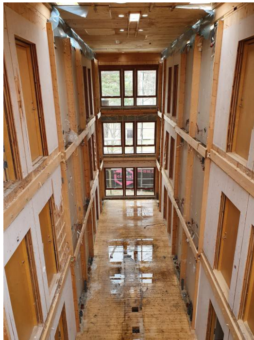
Figure 2 - Space where access balconies previously were.
