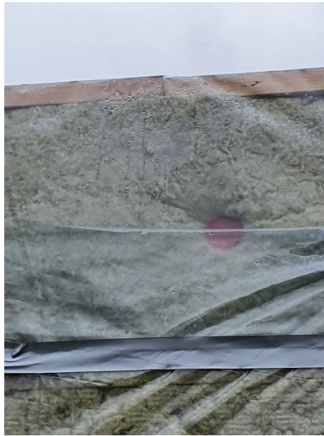
Figure 20 - Condensation inside the plastic.
