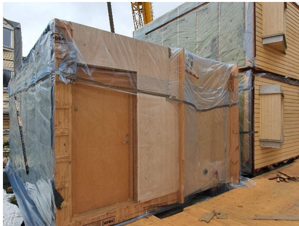
Figure 18 - Wrapped modules waiting for transport.
