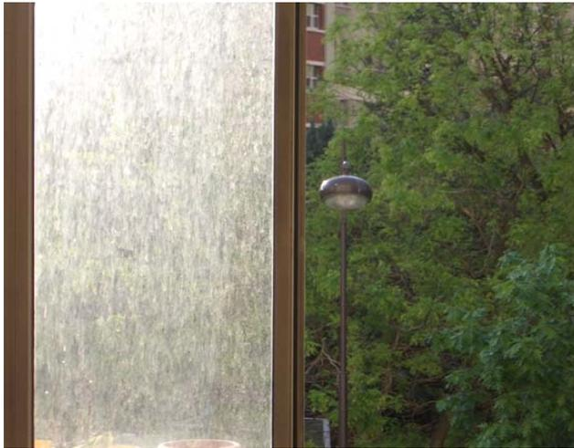
Figure 1.1. Soiling of glass. Detail of a glass window affected by soiling on its left side and opened at the right side
